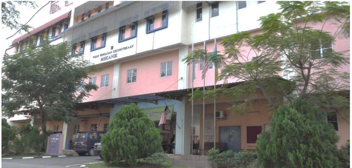
Figure 3.2: The case study building
