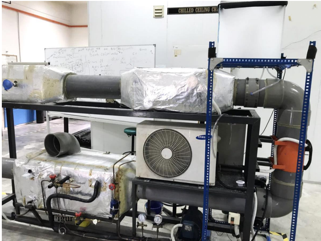
3.9 HVAC experimental rig in Heat Transfer Lab
