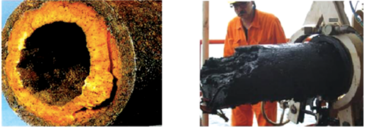
Figure 2. 1 Wax deposition on wall (left) and gelation (right) of waxy crudes in pipeline (Yang et al., 2015)
