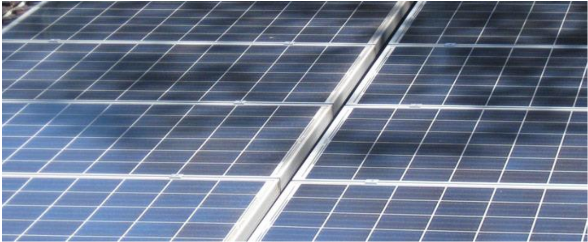
Figure 2.9 Shading due to trees on solar panels which is called as non-uniform shading.
