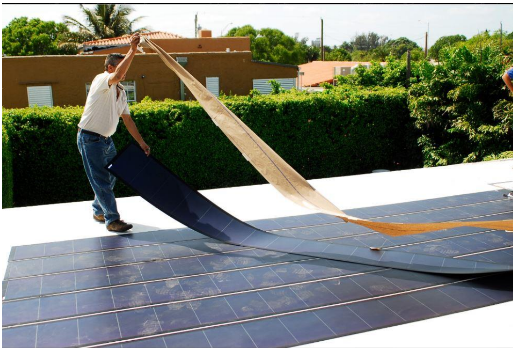
Figure 2.4 : Thin film technologies composed of non-crystalline silicon deposited on a flexible material.
