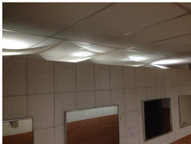
Figure 3.12: Fabric is set up on top of showers' and toilets' stalls
