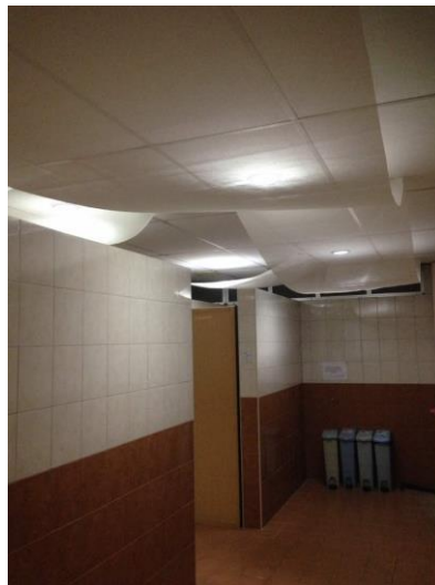
Figure 3.11: Fabric is installed in a wavy-horizontal orientation in the toilet
