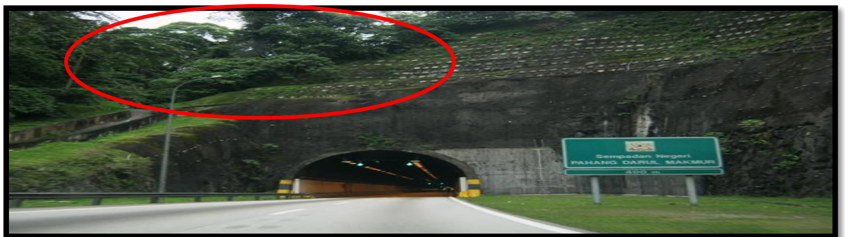
Figure 2.3: Genting Sempah Tunnel located at hill area at Kuala Lumpur-Karak Expressway, Malaysia (Source Nuhu and Maimunah, 2015)
