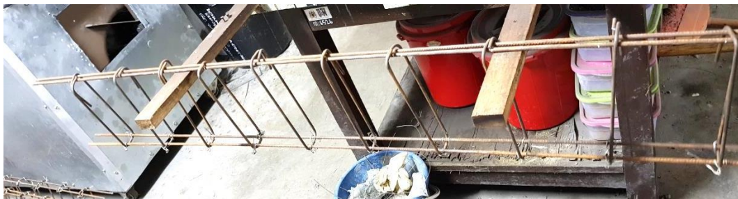
Figure 3.3: Beam reinforcement setup
