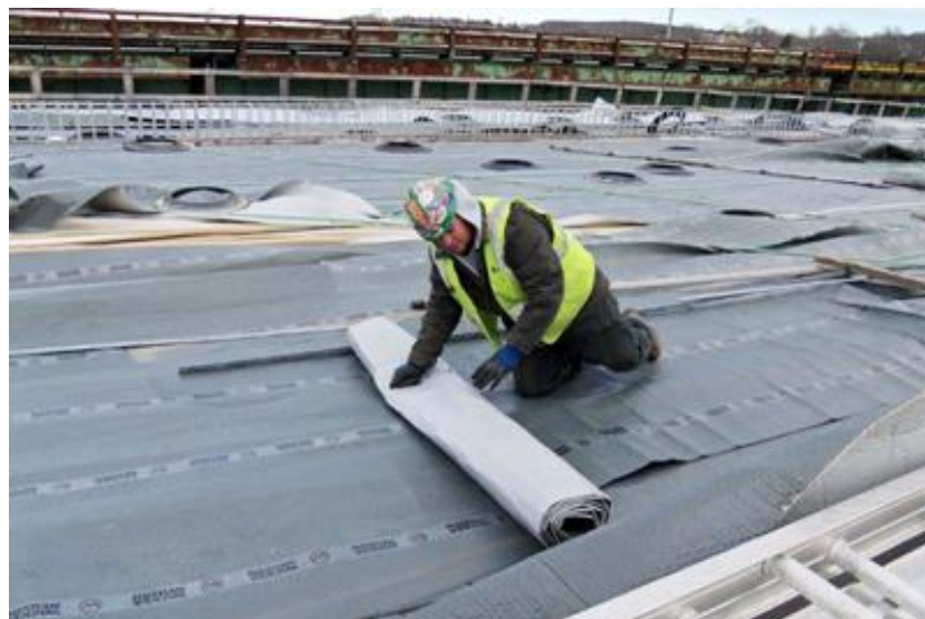
Figure 2.5: Curing blanket used at site
