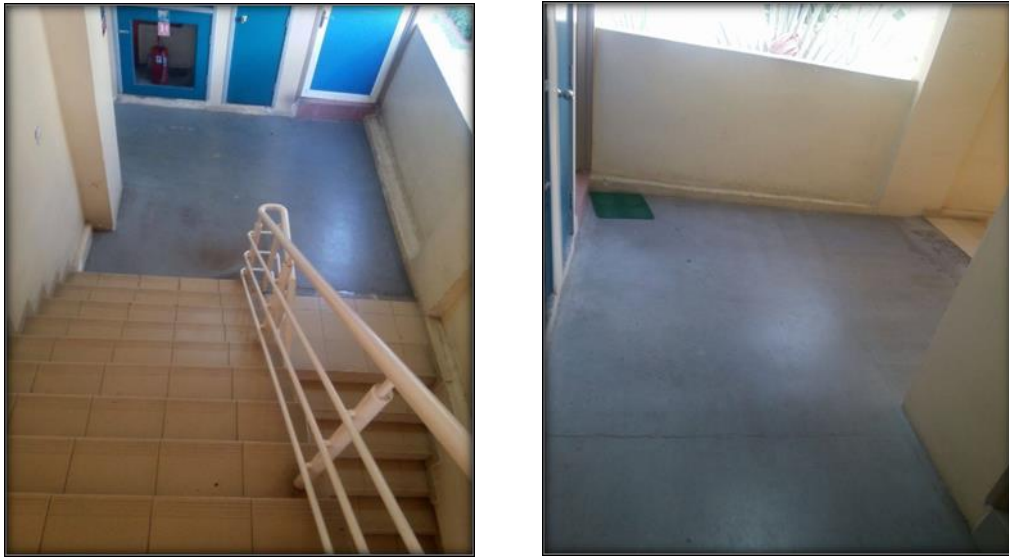
Figure 3.1.2: Angled-walkway at School of Civil Engineering Campus, Universiti Sains Malaysia
