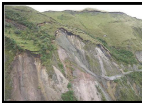
Figure 2.1: Landslide that affected the Pucara Headrace Tunnel.
