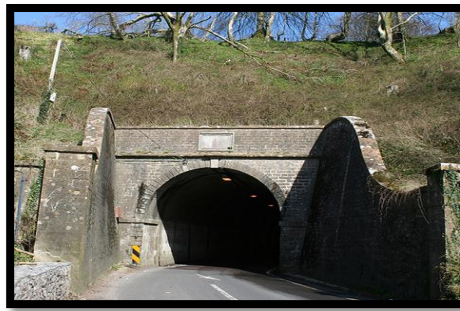
Figure 2.3: Beaminster Tunnel or Horn Hill Tunnel located in England.
