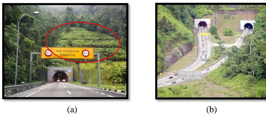
Figure 2.7: Menora Tunnel located (a) at hill area with (b) two-lane highway near Jelapang, Perak, Malaysia
