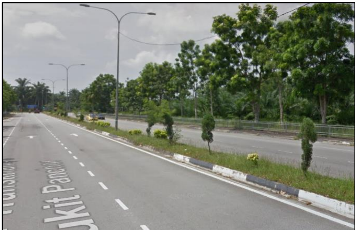
Figure 3.5: Dual Carriageway at Federal Route 282 (Taman Ilmu Indah)
