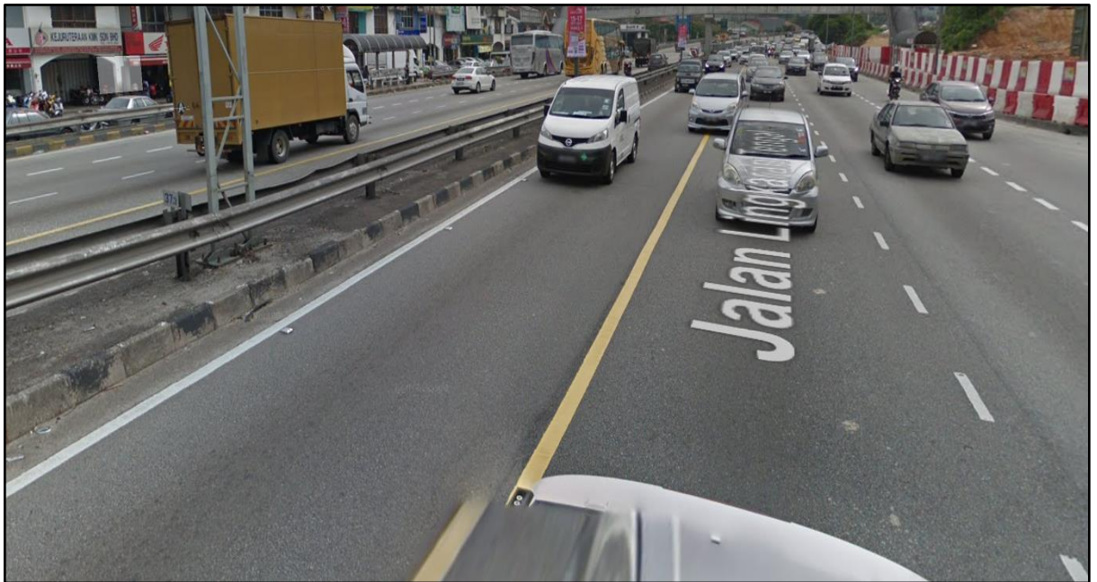
Figure 3.14: Dual-three lane carriageway at BESRAYA Highway
