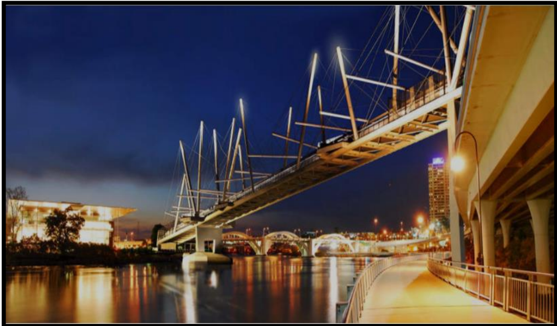
Figure 2.7: The Kurilpa Bridge in Australia completed in October 2009 ( https://www.arup.com/projects/kurilpa-bridge )
