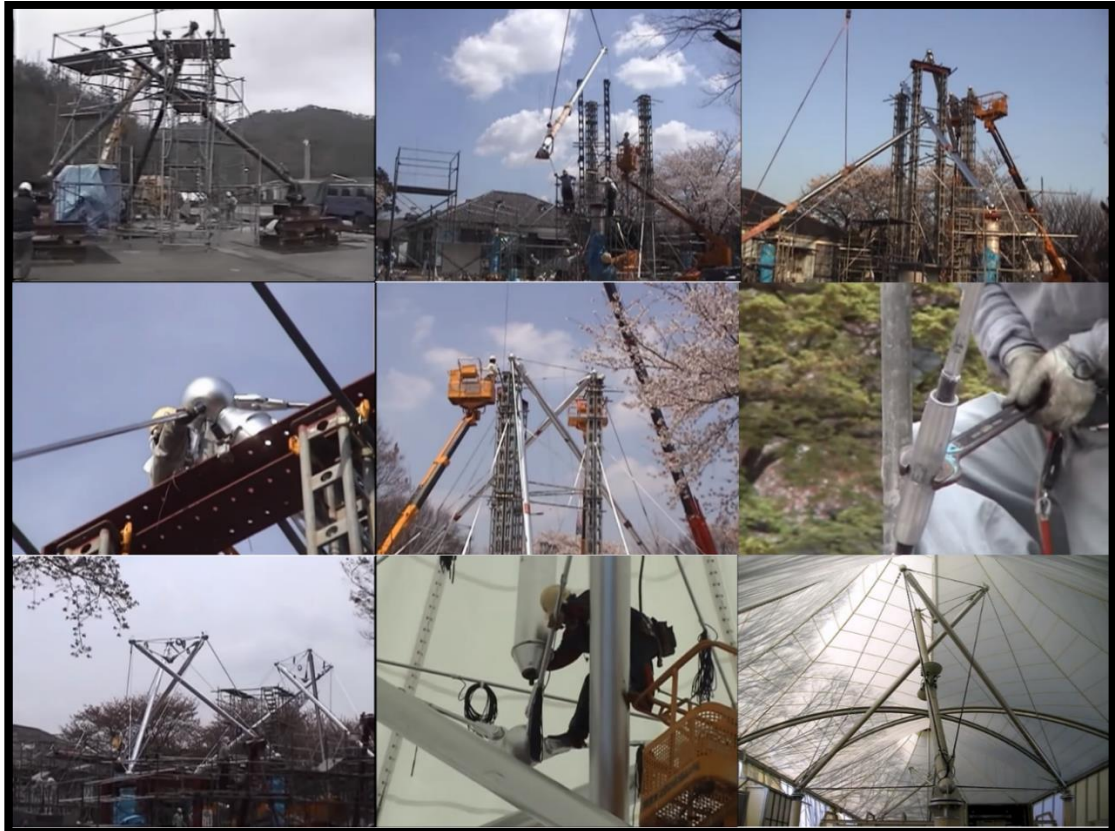
Figure 2.3: Video clippings showing the construction process of the White Rhino ( https://www.youtube.com/watch?v=IeWWPAckC5U )
