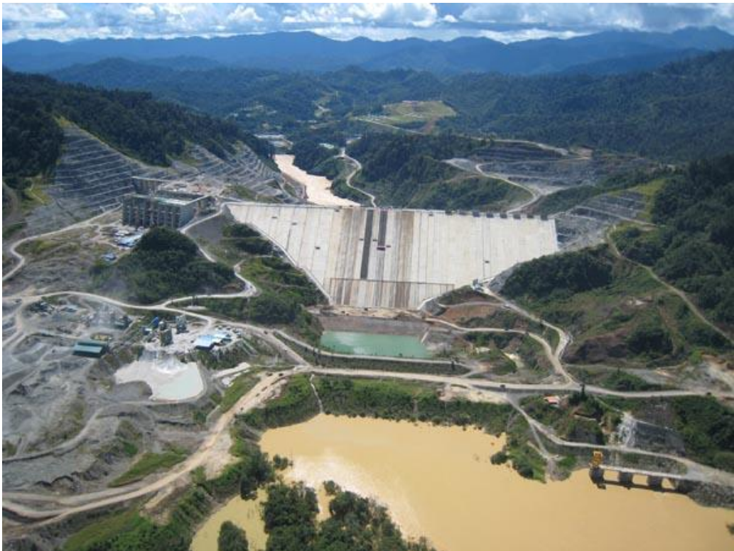
Figure 1.3 Image of Susu Dam (2)
