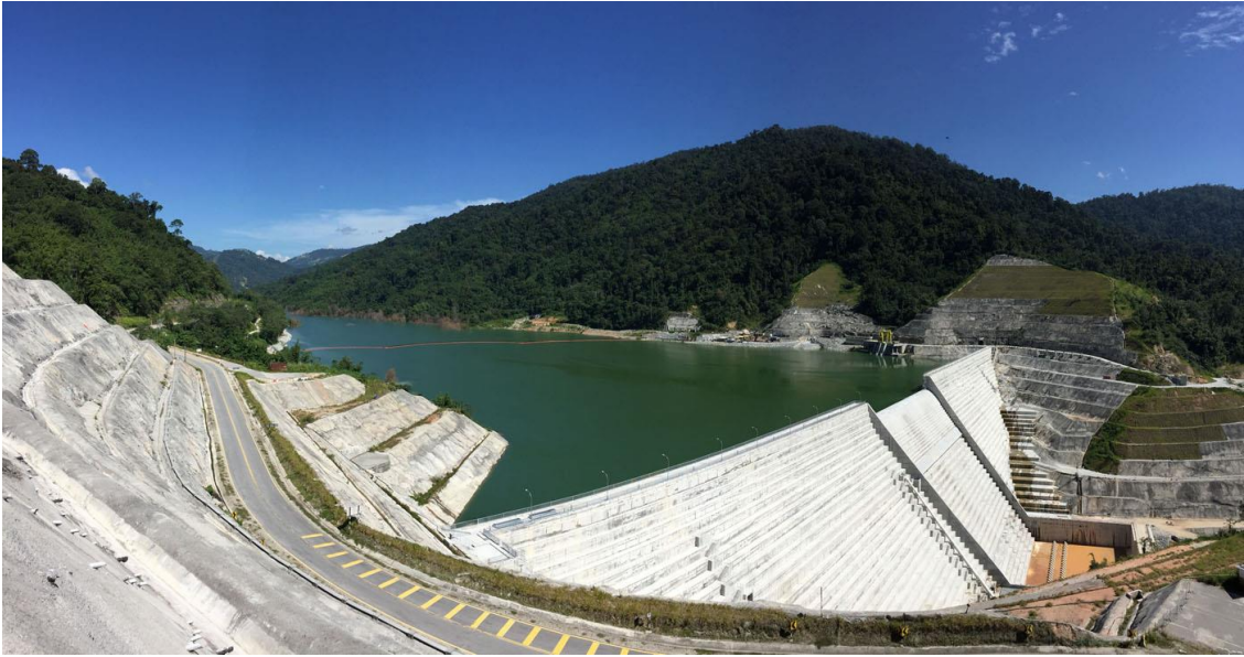
Figure 1.2 Image of susu dam
