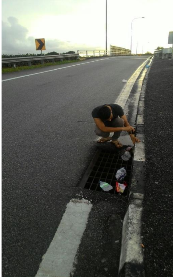
Figure 3.8 Taking the dimension of gully grate
