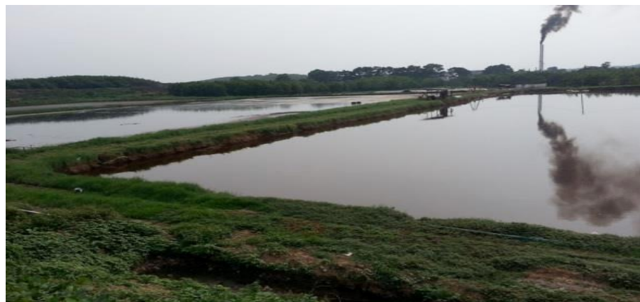
Figure 2.2: Stabilization Lagoon (Ponds) ( Palm Oil Mill Effluent Treatment , 2015)
