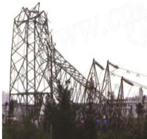
Figure 1.1: Transmission Line Tower collapsed in China caused by wind damage (Jiang et al. 2011).
