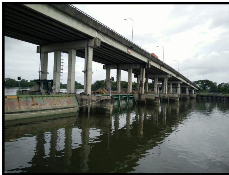
Figure 3.3 : Side view of Sarawak Barrage
