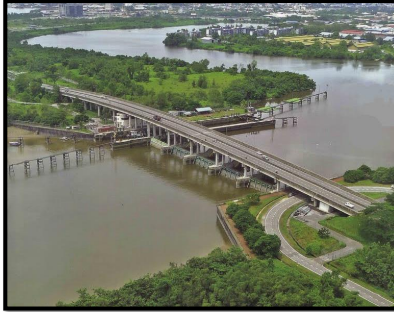
Figure 3.4 : Top view of Sarawak Barrage
