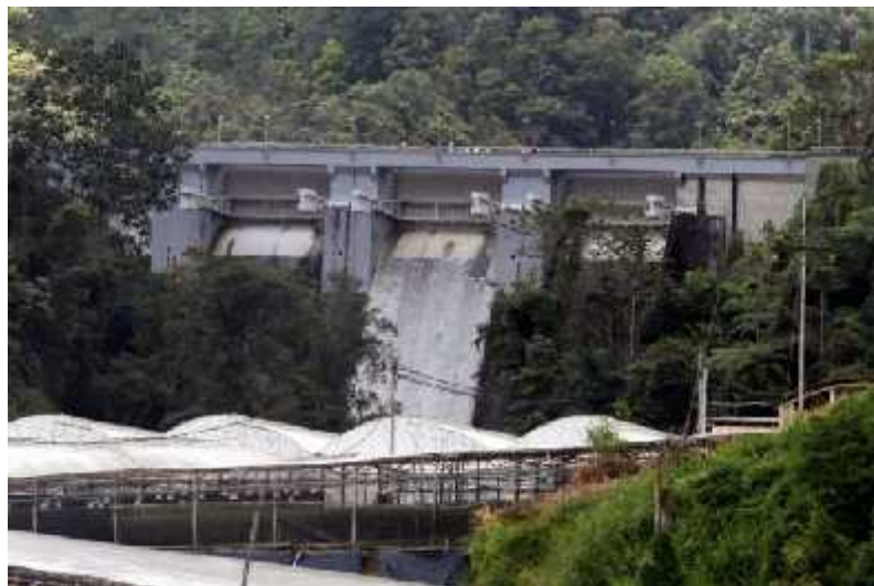
Figure 2.2 : Radial gate at SAB dam
