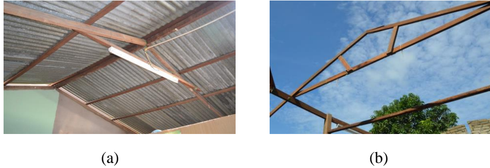
Figure 2.2: View of timber truss system for non – engineered building in rural area showing (a) complete roofing system and (b) bare timber frame (Majid et al., 2016)
