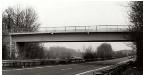
(c) Brücke Hesseler Weg Bridge, Germany (The first prestressed concrete bridge) (Sigrist and Baurich, 2006)
