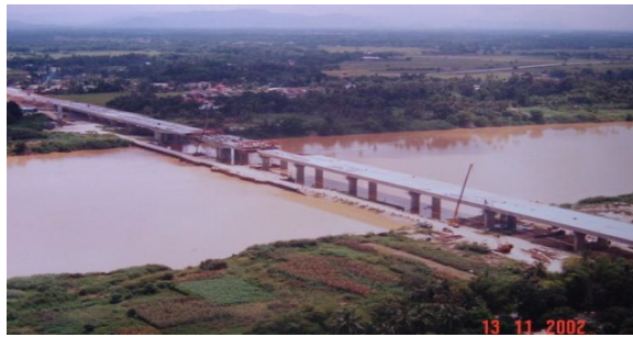
(b) Sungai Kelantan Bridge, Malaysia (Giga Engineering & Construction, 2001)
