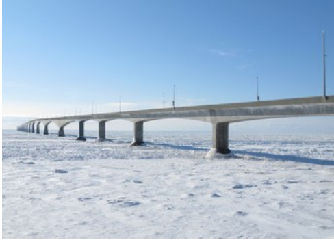
(a) Beam bridge: Confederation Bridge, Canada
