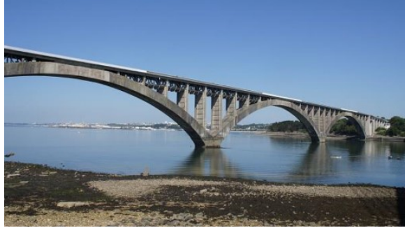
(a) Plougastel Bridge, France (Structurae, n.d.)
