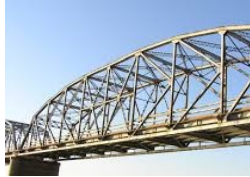
(b) Truss bridge: Arun Khola Bridge, Nepal
