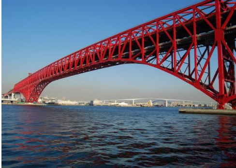
(e) Cantilever bridge: Minato Bridge, Japan
