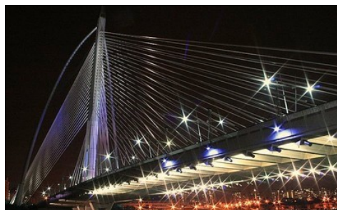
(g) Cable-stayed bridge: Sri Wawasan Bridge, Malaysia
