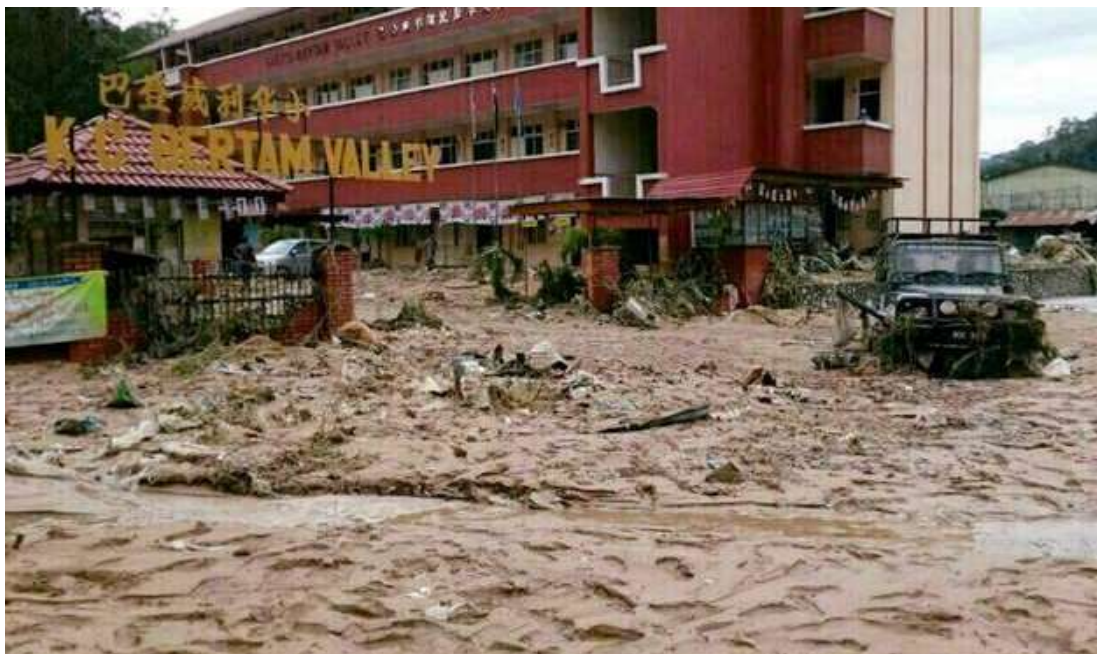
Figure 1.1: Mudflow Disaster in Cameron Highlands (Yong, 2013)
