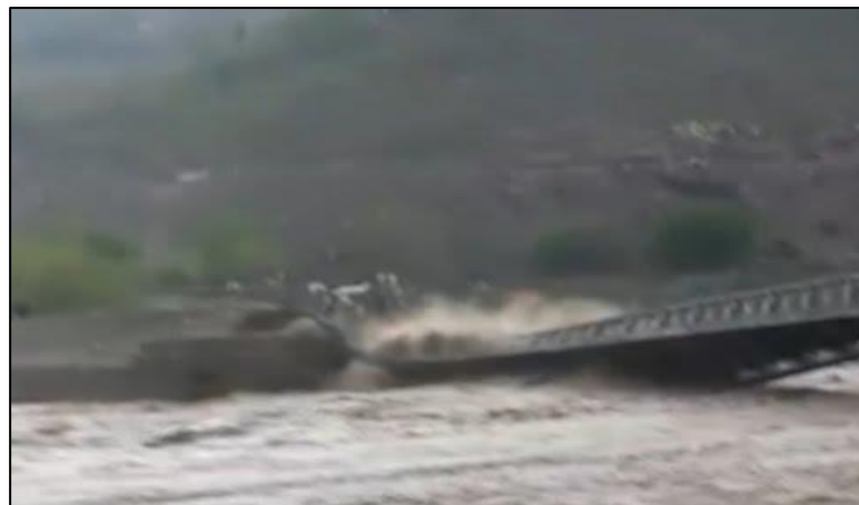
Figure 1.4: Bridge Collapse During the Flood Event in Lower Dir (BBC, 2016)
