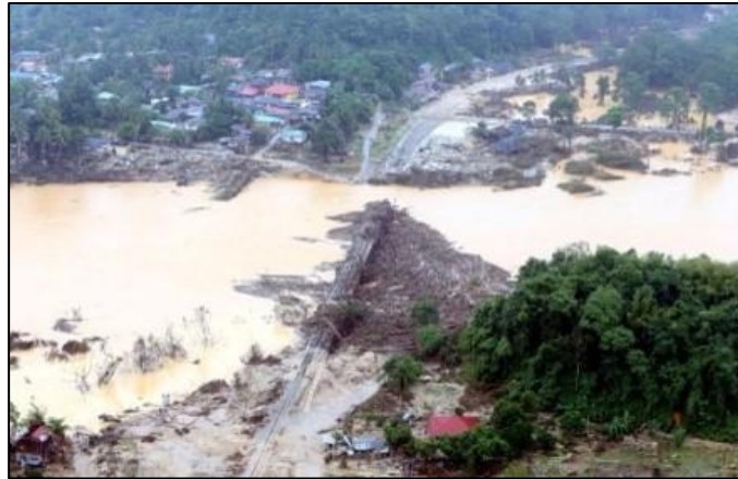
Figure 1.2: Debris Accumulated at Bridges in Kelantan During the Recent Flood (Straitsimes, 2014)
