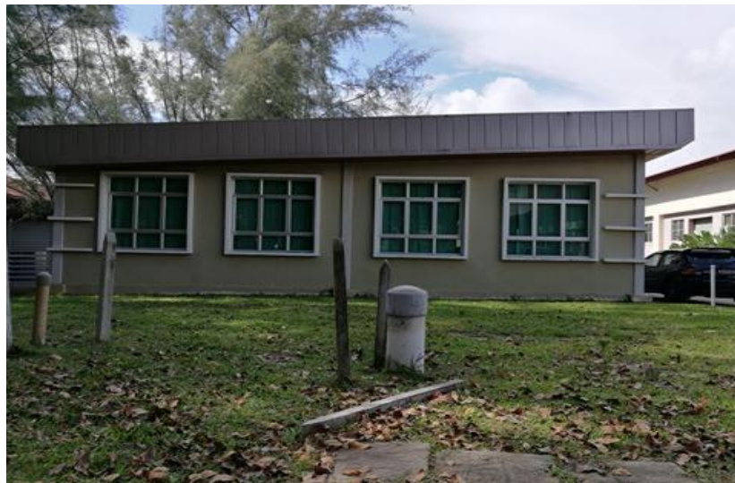
Figure 3.2: USM Groundwater Tube Well
