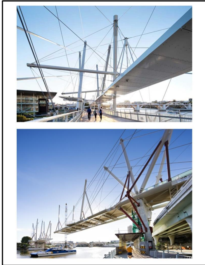
Figure 2.3: Kurilpa Bridge and self-supporting during construction stage (Source: http://www.coxarchitecture.com.au )
