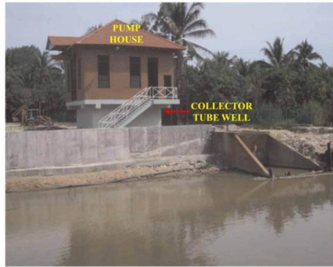
Figure 2.3: RBF at Wakaf Bunut water treatment plant, Kelantan, Malaysia (Sources: Chew et al. , 2015)
