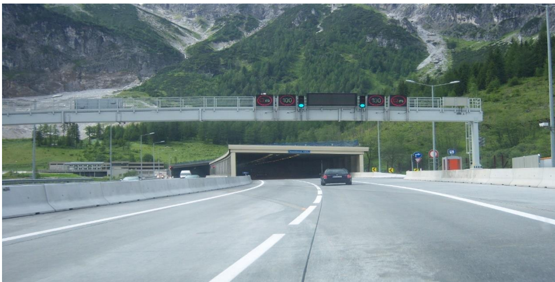
Figure 2.10. Tauern Tunnel (Source: Kim et al., 2010).
