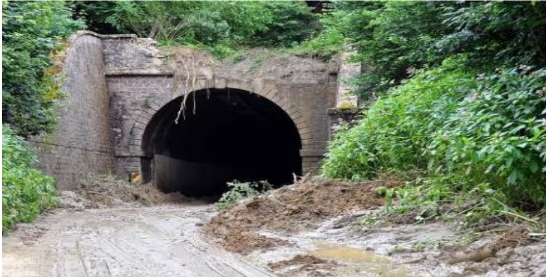
Figure 2.9. Beaminster Tunnel (Source: Andrew, 2012).
