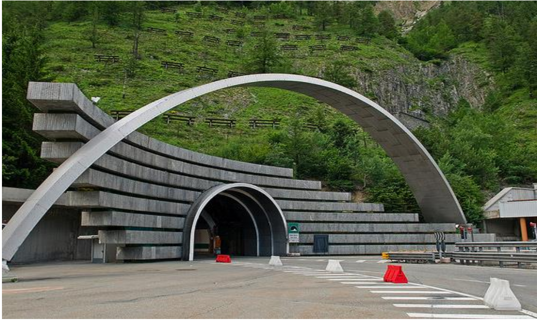
Figure 2.4. Mont-Blanc Tunnel between Italy and France (Source: Leonelli et al., 2012).
