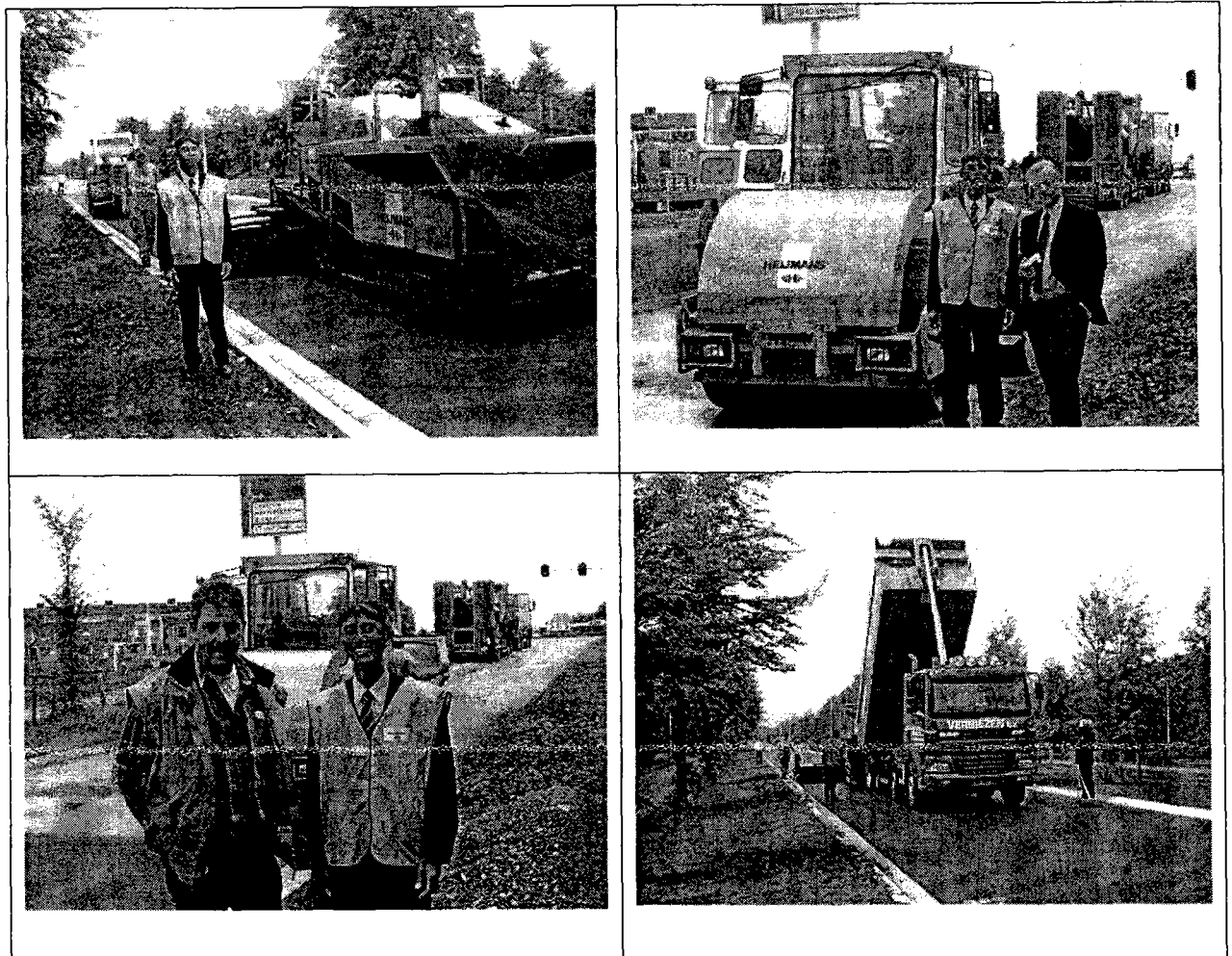
Figure 9 Thin Surfacing Construction Near Eindhoven
