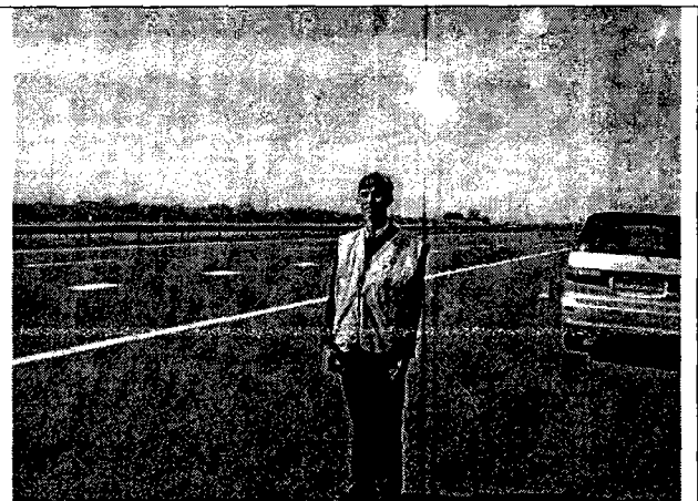
Figure 6(b) Highway Section Paved with Rubberised DLPA
