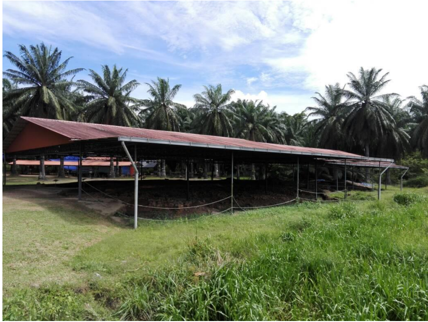
Figure 1.5: An open-air roof structure with safety rope at site SB2B & SB2D.
