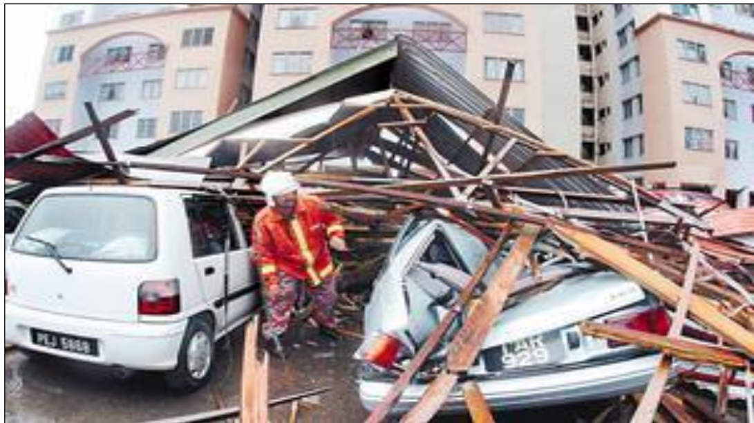
Figure 2.1: Roof Structures of an Apartment Landed on top of Vehicles (Archive (Utusan, 2004))
