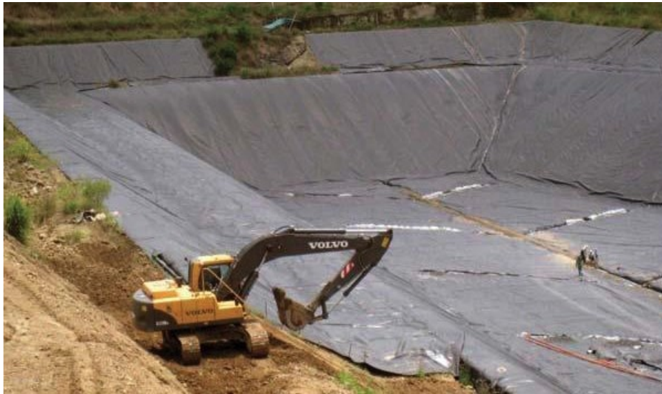
Figure 1: The landfill while being prepared
