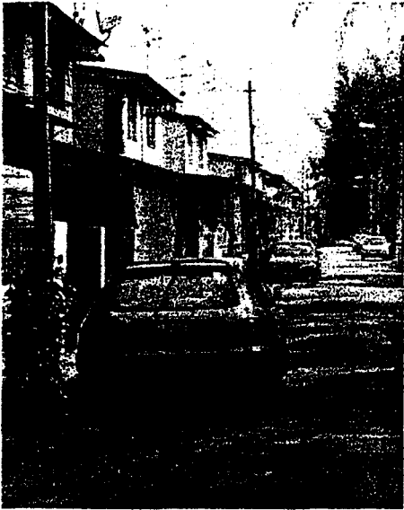
Cluster housing at Sungai Pinang
