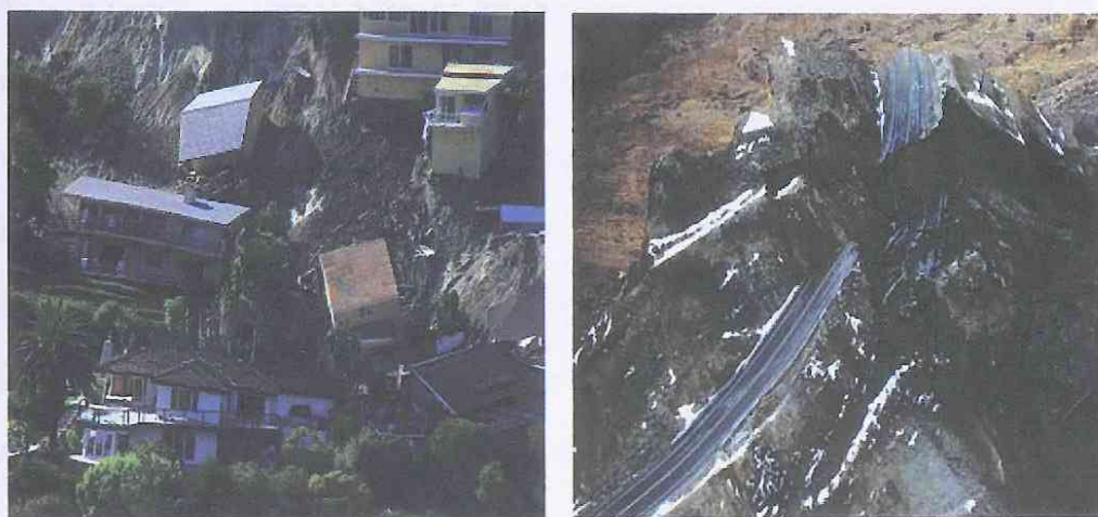
Figure 2.1: Damages caused by landslides (Google source, 2013)
