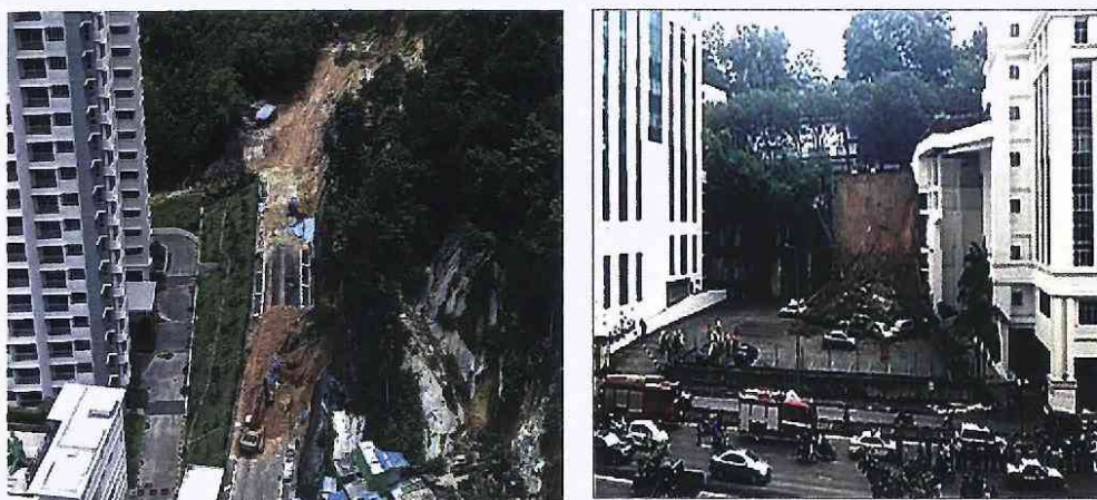
Figure 1.1: Damage caused by landslide at Penang Island (Google source, 2013)
