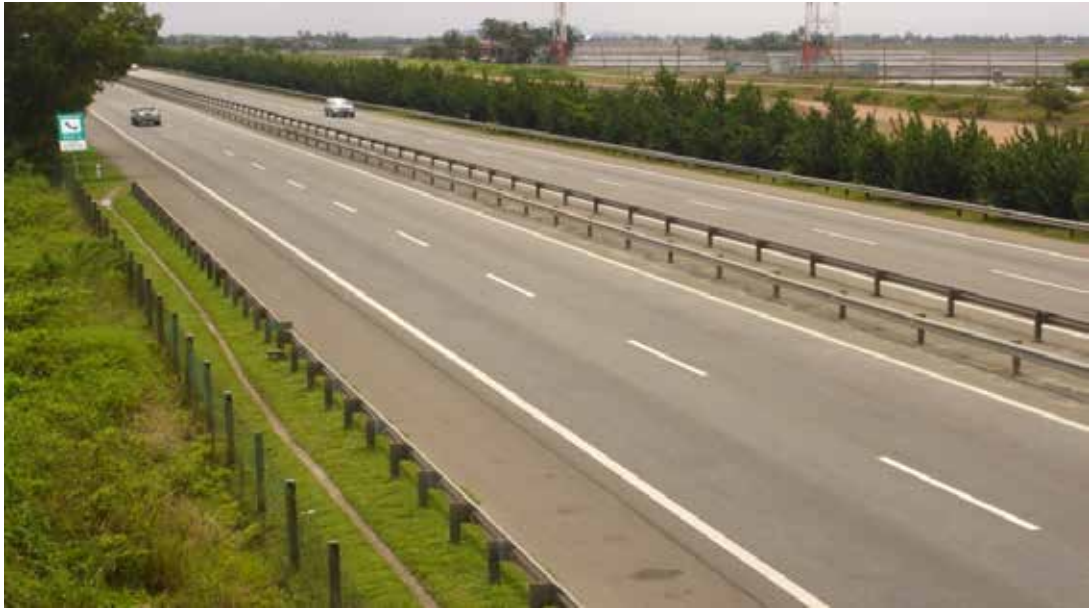
Plate 1.1: Typical 4-lane basic segment expressways in Malaysia
