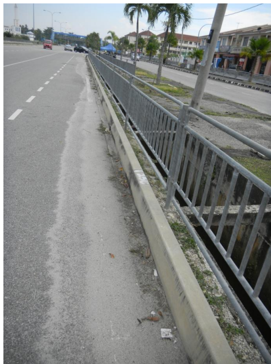
Figure 2.1: Sand and aggregates from road surface material accumulating by the roadside which will be washed into roadside open drain when rains
