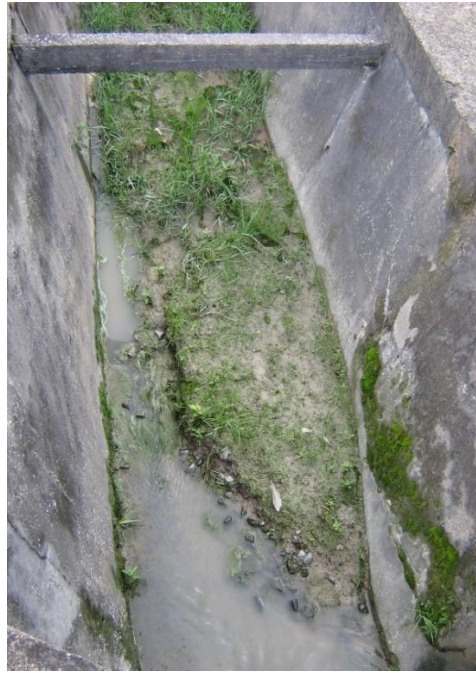
Figure 1.1: Sediment deposition in open concrete drain
