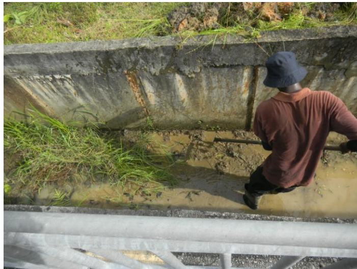
Figure 1.2: Removing sediment deposition in open concrete storm drain manually
