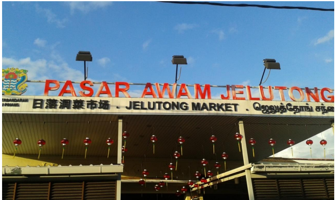
Plate 1.1 Jelutong wet market building
