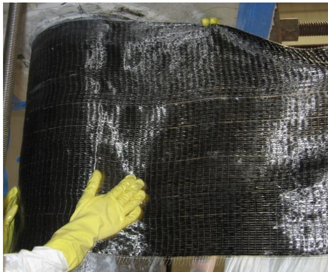
Figure 1.4: Repair of damaged bridge columns using Fibre Reinforced Polymer ( http://cceer.unr.edu/projects/repair_of_bridge_columns/nhs2r.html )
