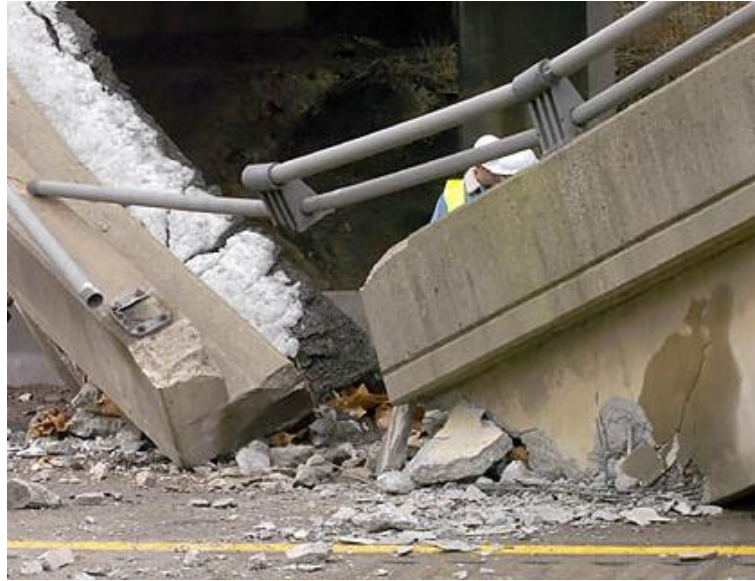
Figure 1.1: Partial collapse of the exterior girder of an overpass caused by pre-stressed reinforcement corrosion due to the application of deicing salts (Grata, 2005)
