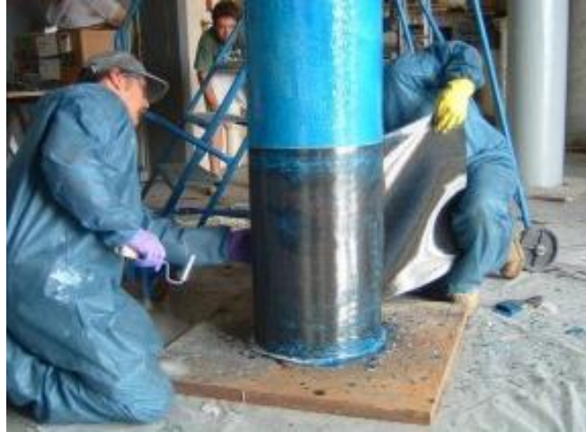
Figure 2.7: Installation of FRP reinforcement ( http://www.compositesmanufacturingblog.com )
