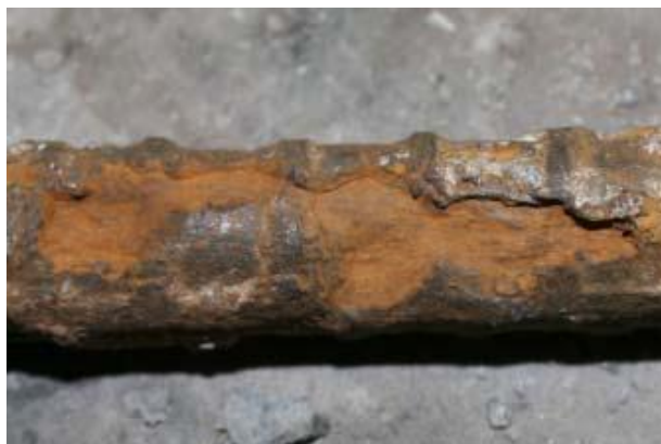
Figure 2.2: Pitting corrosion in steel reinforcing bar by chloride attack (Parish, 2008)
