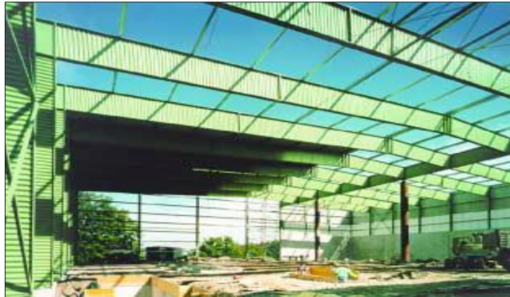
Figure 1.1 The corrugated web I-beams for both columns and girders (Zeman and Co, 1999)
