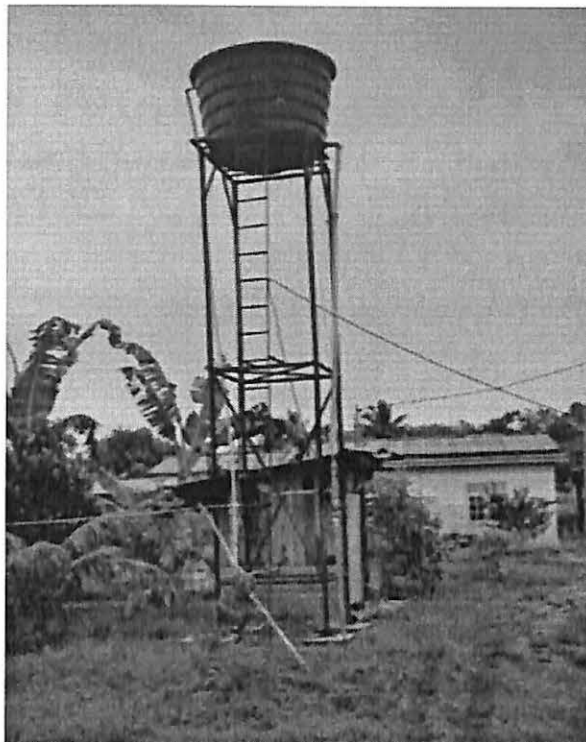
Photograph 1: Tube well with over-head tank water system
