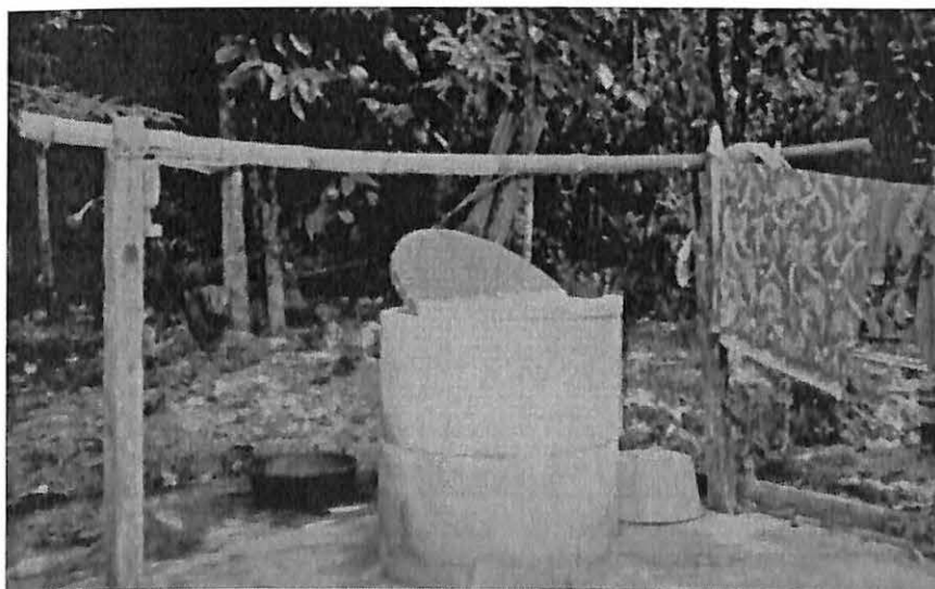
Photograph 2: Open dug well with direct connection water system
