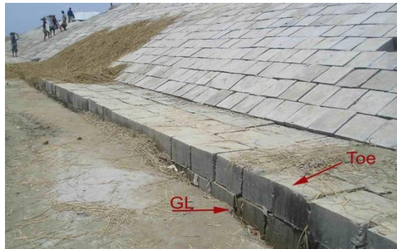
Figure 17. Toe structure above ground level Source: Research.
