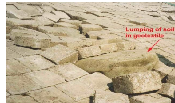
Figure 18. Lumping of soil in the geotextile due to wave suction Source: Research.
