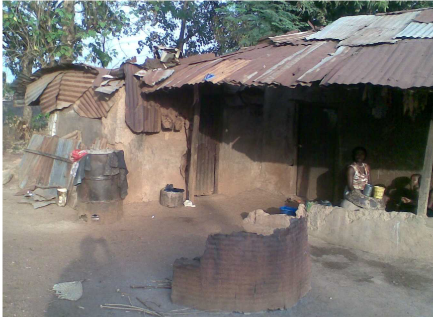
Figure 3. House with Rendered Clay Block Walls
