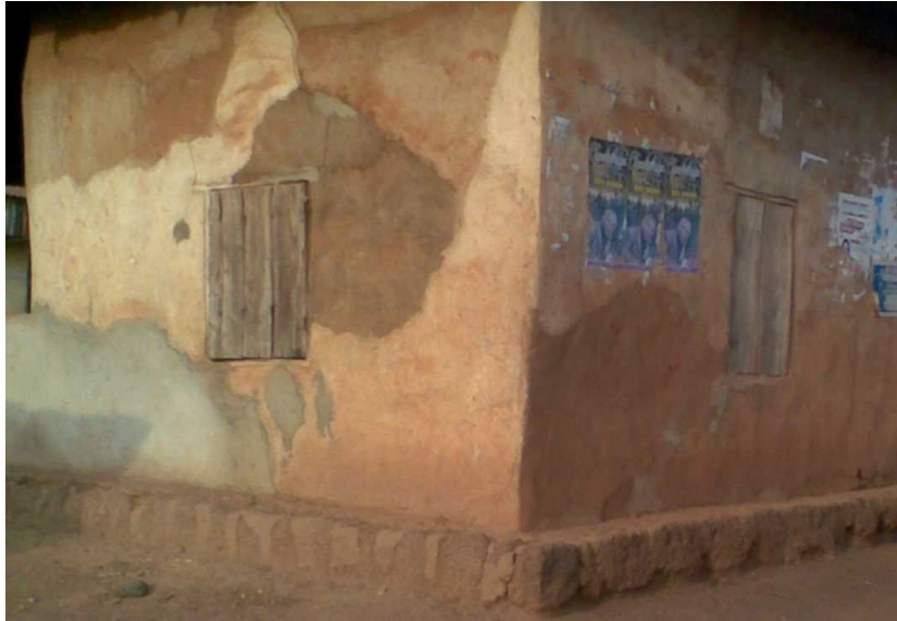
Figure 5. House with Timber Boards over Openings
