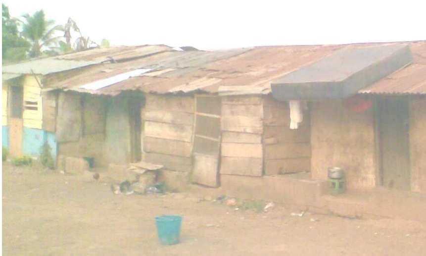
Figure 4. Houses with Reclaimed Timber Boards as Walls
