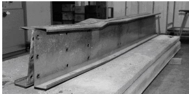
Figure 2. Failure in Channel-Sections as Influenced by the Length of the Bolt-Group (Lim and Nethercot, 2003)
