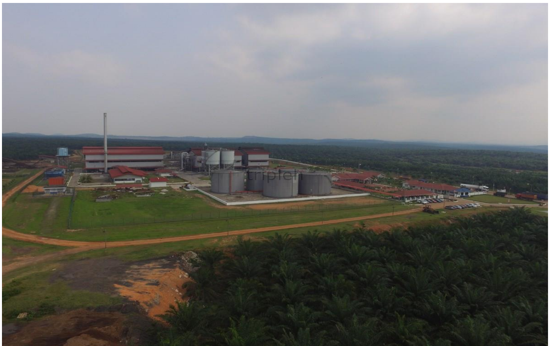
Figure 2.1. Typical palm oil mill at Sime Darby Plantation - KKS Sua Betong, Port Dickson, Negeri Sembilan.
