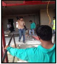
Figure 3. Workers not wearing any (PPE) during construction work.
