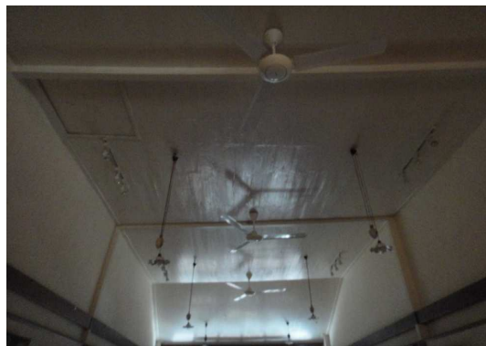
Figure 5. The ceiling of the first floor free from defects
