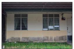
Fig. 2: Peeling paint on external wall
