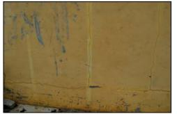
Fig. 1: Vertical and horizontal cracks on outer wall
