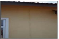
Fig. 3: Vertical cracks on external wall
