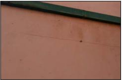
Fig. 5: Plaster cracks on external wall
