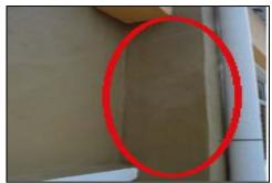
Fig. 4: Diagonal cracks on column area
