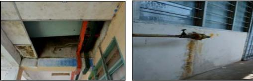
Fig. 9: Broken suspended ceiling
