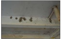
Fig. 7: Concrete spalling on beam area
