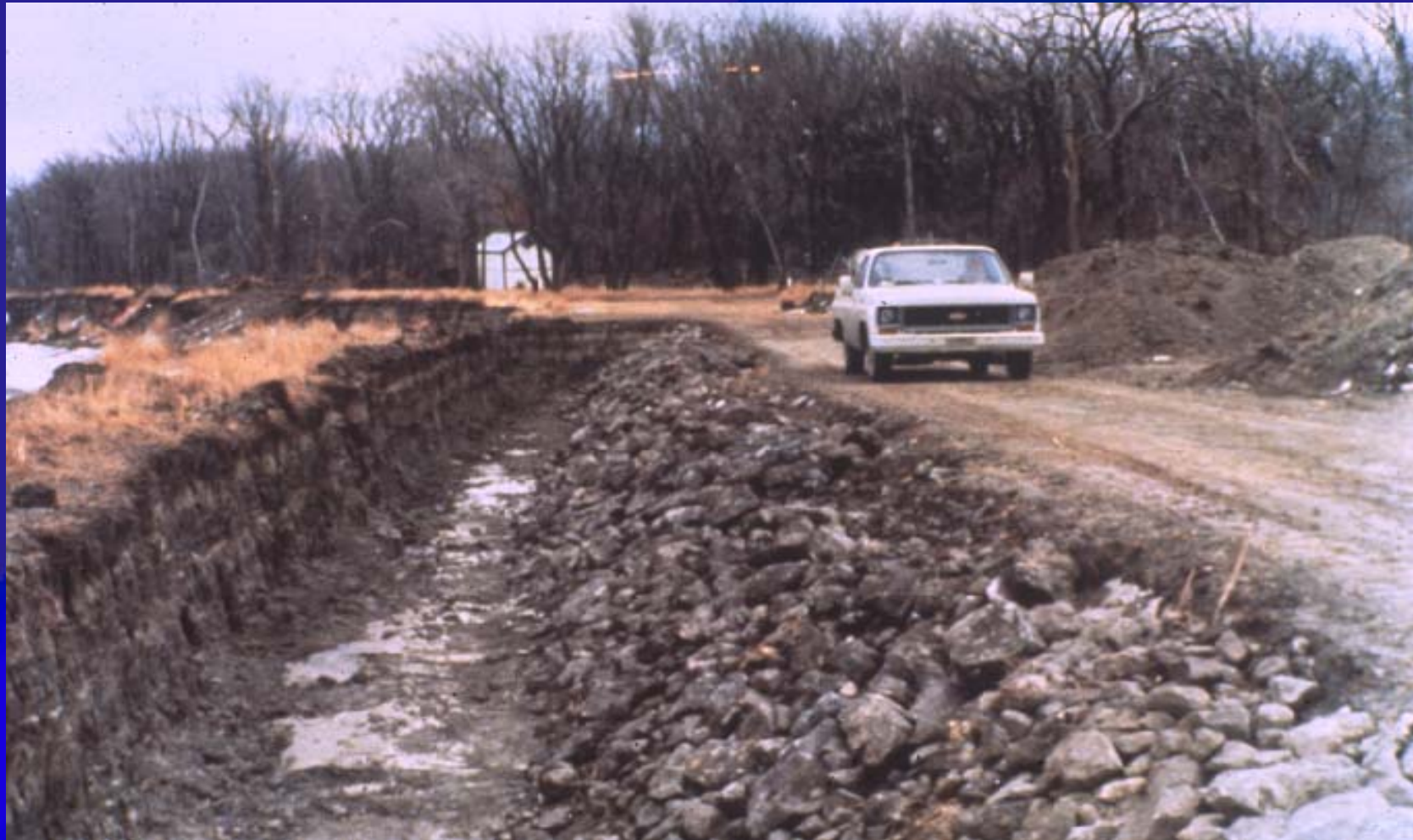
Figure 7.5 Placement of Windrow Debris Enclosed Through Top Deck
