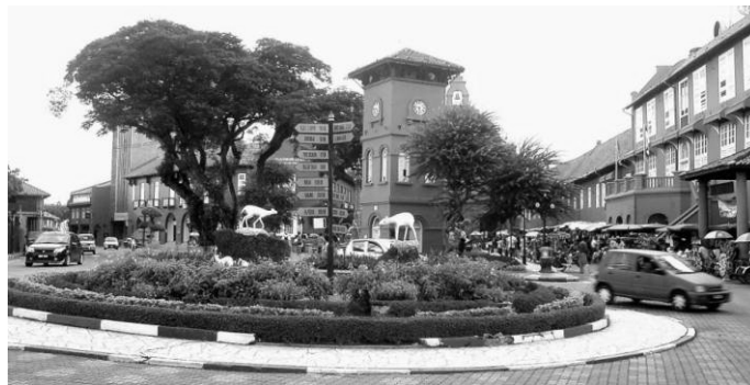
Figure 3: The red building is always referred as landmark due to its colour and architectural styles which is contrast from the surrounding.
