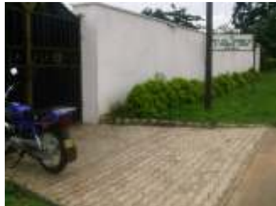
Plate 5.15: Use of interlocking stones for Demarcating flooring with colours
