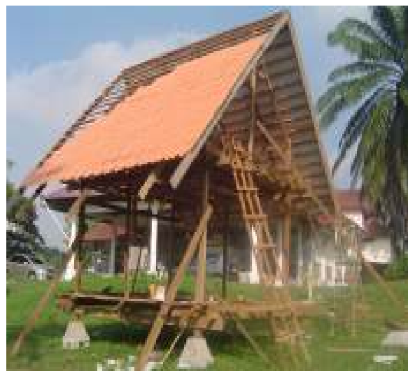
Complete module of the house
