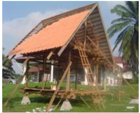
Preparing the roof covering material
