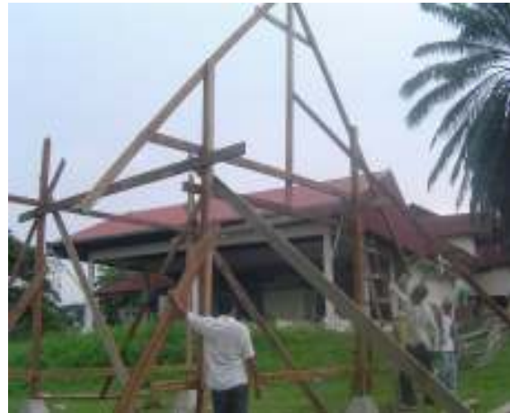
Erecting the main structure
