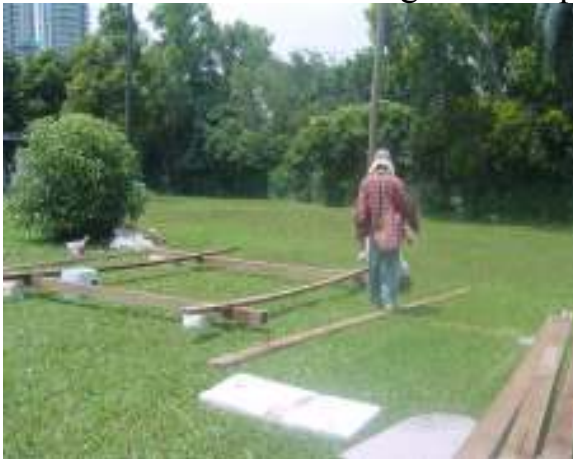
Preparing the site
