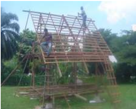
Completing the roof structure
