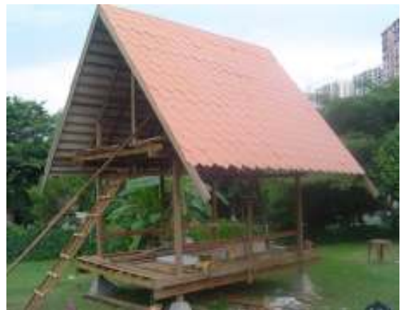
Partially completed house.
