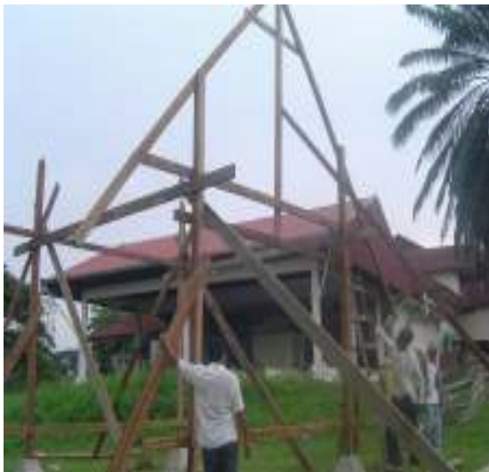
Erecting the first panel of superstructure.
