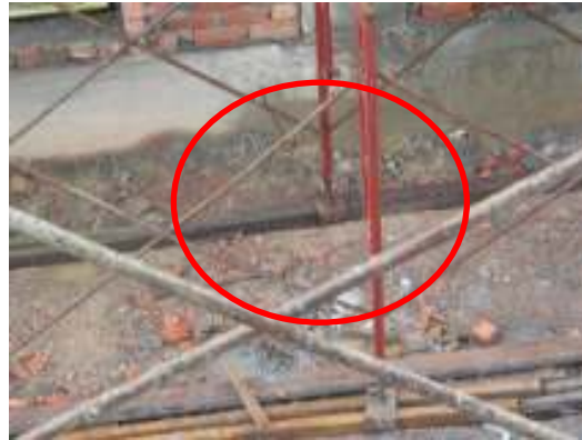
Figure 1 :Good condition of footing scaffolds at Bungalow Project,
